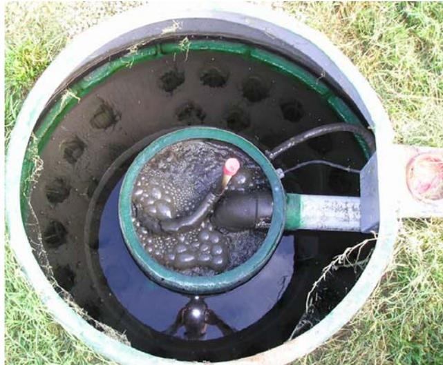
**Figure 5—Enviro-Guard Treatment Tank at NSF Test Facility**
