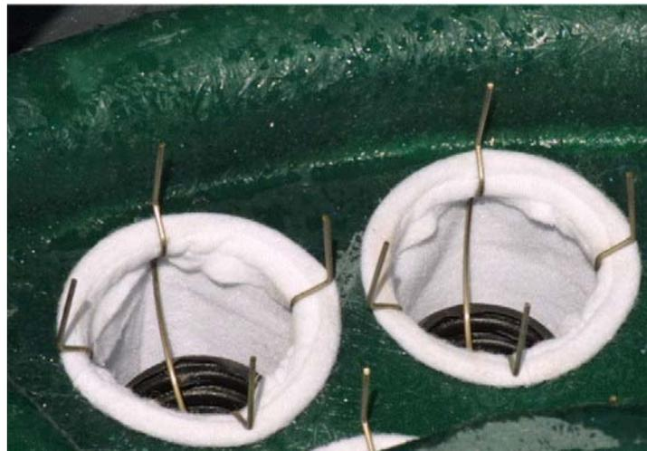
**Figure 4—Fixed Film Media and No-Bypass Weir Plate**
